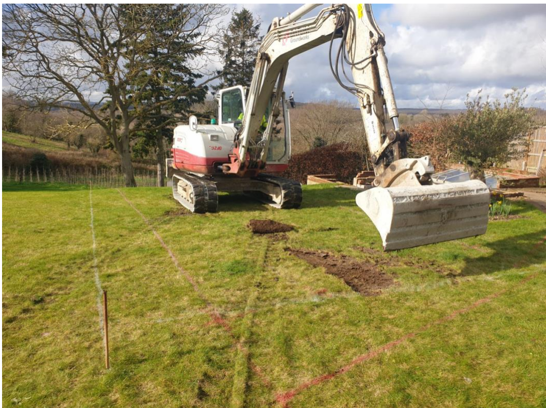
Plate 2, Working shot of turf removal by 9t excavator with 1.5m ditching bucket
